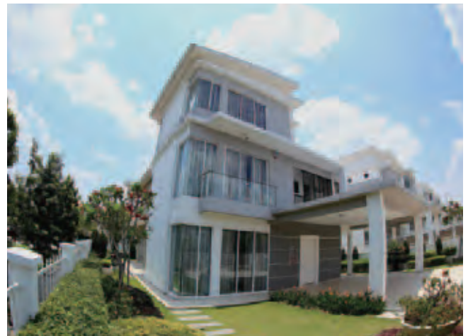
Bungalow units at Urbana @ D'Alpinia, Puchong
